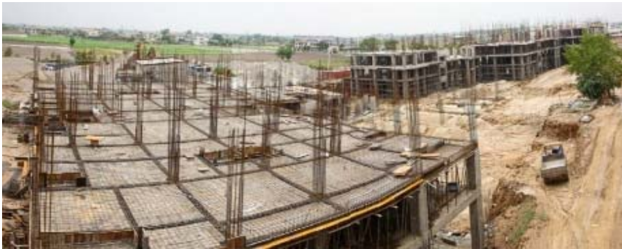
(Towers under construction i.e. J, K, L, M and N)
